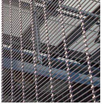
(06) MS: MESH SCREEN **ALUMINIUM MESH POWDER COATED DARK GREY**
