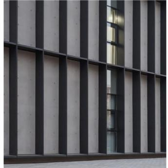
(07) ALS: ALUMINIUM LOUVRE SCREEN **VERTICAL ALUMINIUM** SUNPROTECTION SCREEN WITH DARK GREY PAINTING
